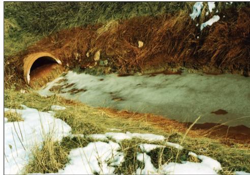
Photo 3. Foamy alkaline water flowing out of leakage of sludge reservoir (Photo by JUHÁSZ, Á. 2003)
