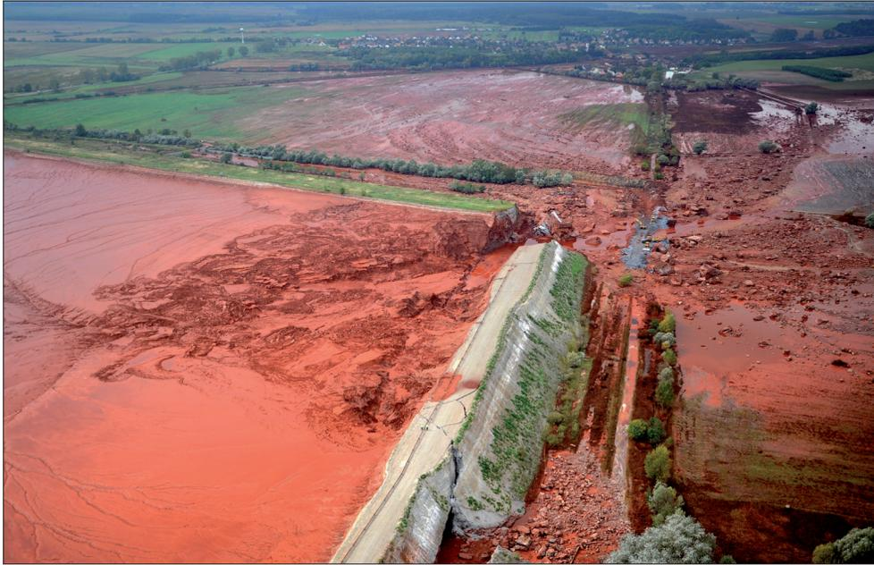
*Photo 1.* Damaged dam of cassette No. 10 and areas affected by the red sludge flood. (Photo by H. SZABÓ, S. MTI)
